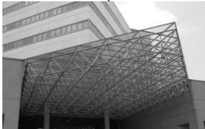
Figure 4 : architectural illustration of truss structure.
