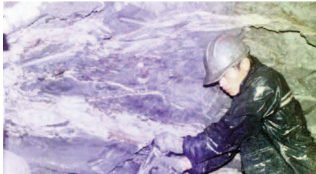
TAIWAN - Tunnel de Tzechiang
